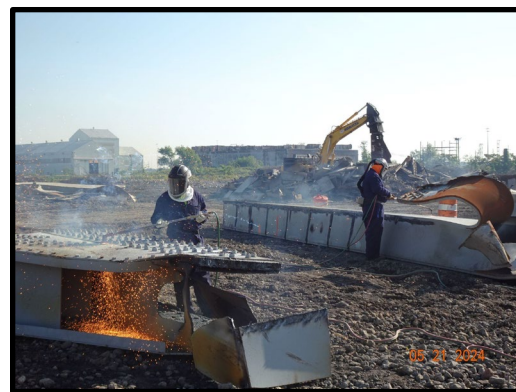
Photo 1 shows two employees wearing coveralls and PAPR's using 5 foot long torches to cut sections of bridge.
